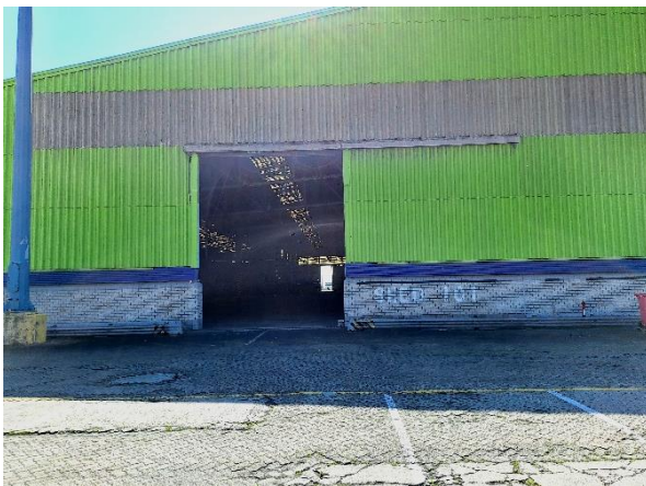
Figure 8: Shed 101 - Outside View
