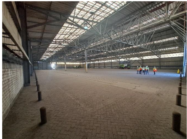
Figure 9: Shed 101 - Inside View
