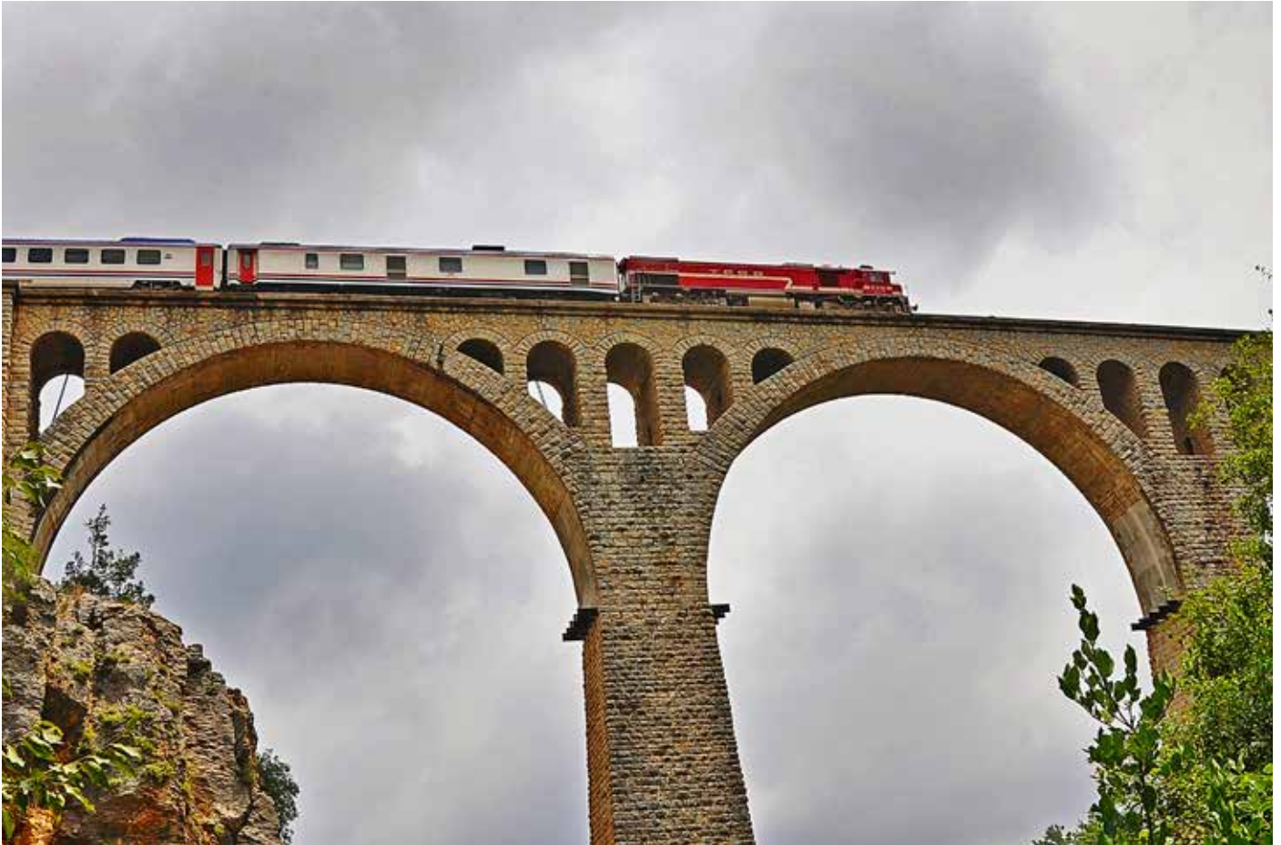
Varda Bridge / Toros Express
